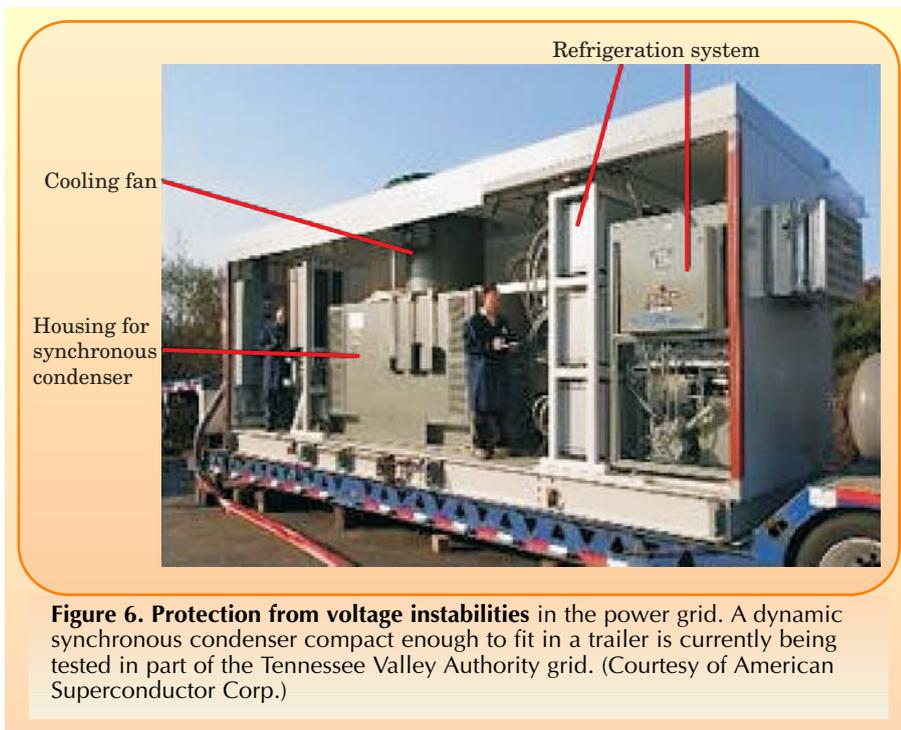
**Figure 6. Protection from voltage instabilities** in the power grid. A dynamic synchronous condenser compact enough to fit in a trailer is currently being tested in part of the Tennessee Valley Authority grid. (Courtesy of American Superconductor Corp.)
